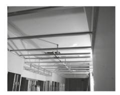
Shortspan grid and Locking Angle Trim make drywall framing faster and easier
